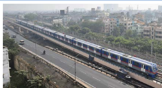
Metro viaduct to embankment
